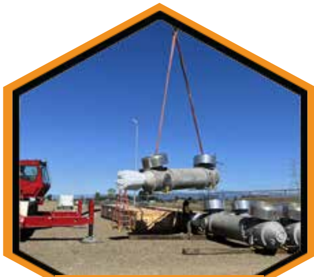
Supply & Delivery of 550KV dead pole breakers to customer site
